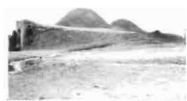
Raised entrance and the domes over the changing and bathing rooms are the only visible part of many traditional beths. Baths are below ground level for insulation and to allow water supply to flow by gravity.
